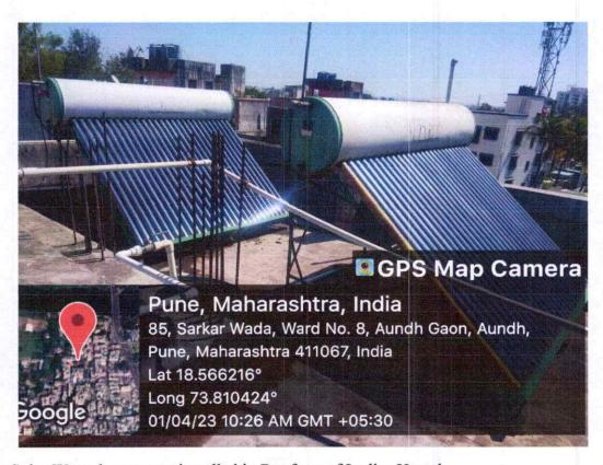
Two Solar Water heaters are installed in Roof top of Ladies Hostel.
