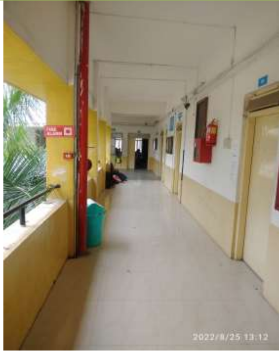
Properly placed dust bins in college for waste disposal
