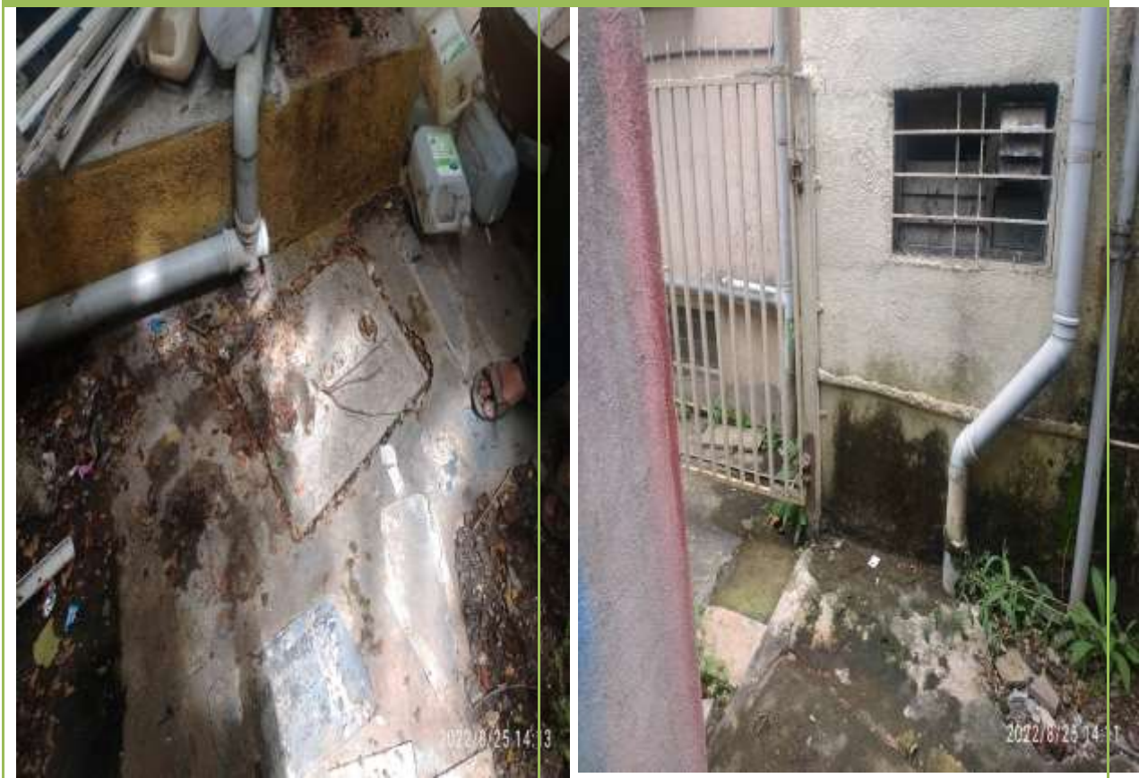
Rain water harvesting system in college premises
